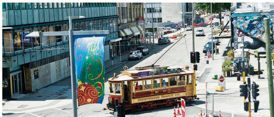
The BNZ Centre courtyard forms part of the Stage II development that is currently under construction.
